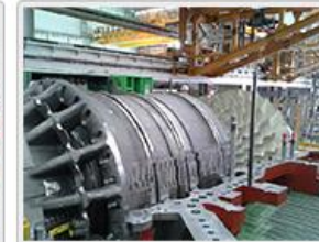
Blade Ring Dismantling, Lifting
